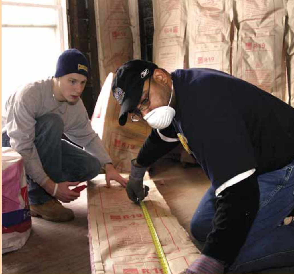
Daniel Theal '08, co-president of the Canisius Chapter of Habitat for Humanity, and David Burton measure and trim insulation for one of the four bedrooms.
