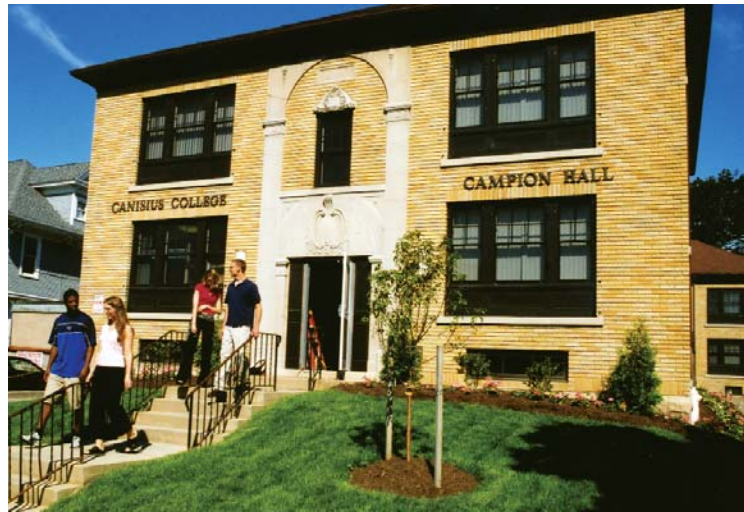
Campion Hall, home to the college's new Intercultural Living Center, is located on Main Street between Kensington and Dewey avenues.
