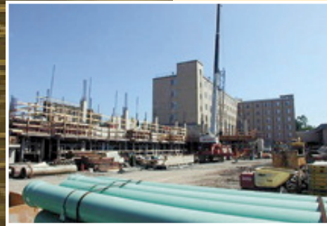
PHOTO (LEFT): Frisch Hall Construction- October 7, 1962 Photo courtesy of Canisius College Archives
