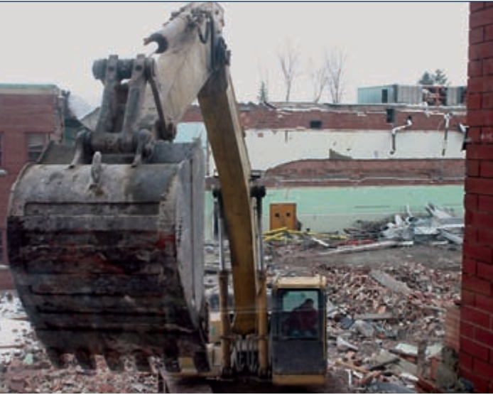
Demolition of the former Mount St. Joe's Academy began on January 14.
